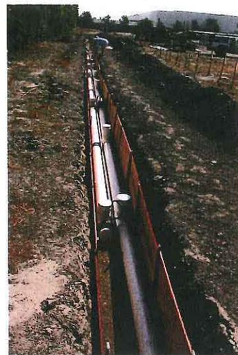
Horizontal Extensometer Construction
